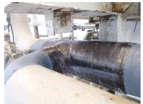
Above: Belzona SuperWrap II tackles complex geometries
